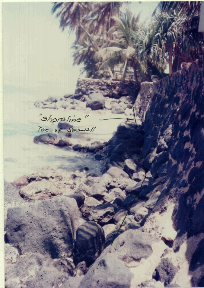
"Shoreline" is the toe of Seawall. Photograph taken at south side of property looking north on 5/28/86
