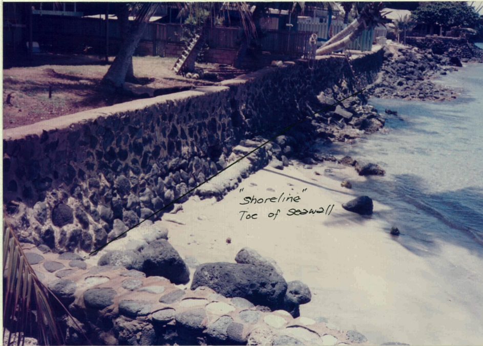
"Shoreline" is the toe of Seawall. Photograph taken at NW corner of property. 5/28/86
