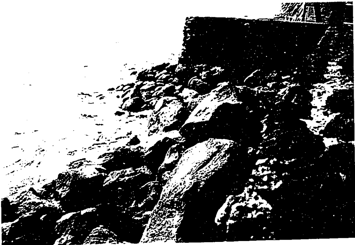
Photograph - 4 View of Shoreline/Seawall
